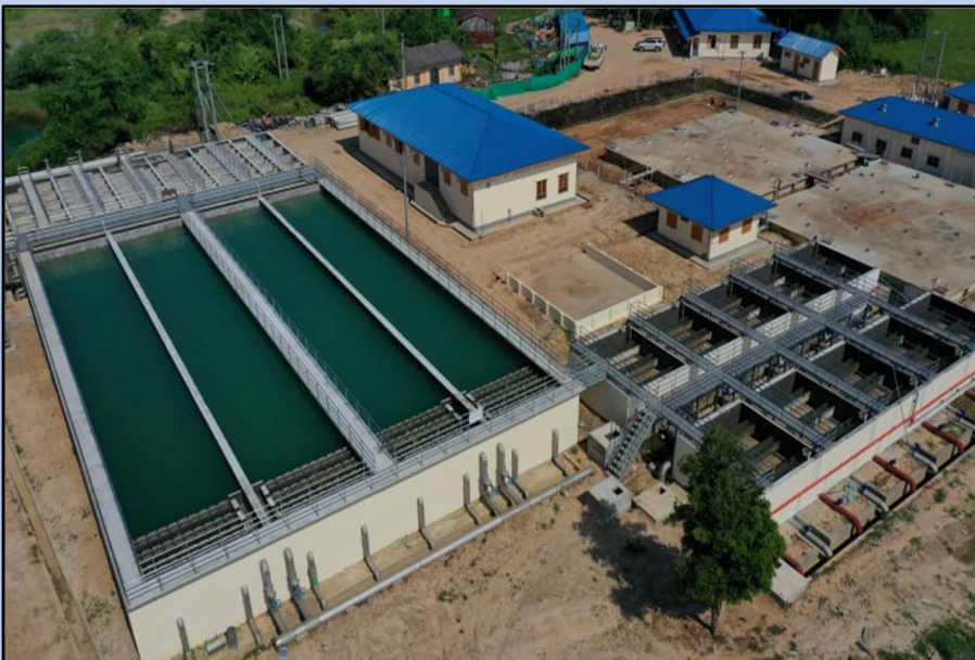
Sedimentation tank and RSF
