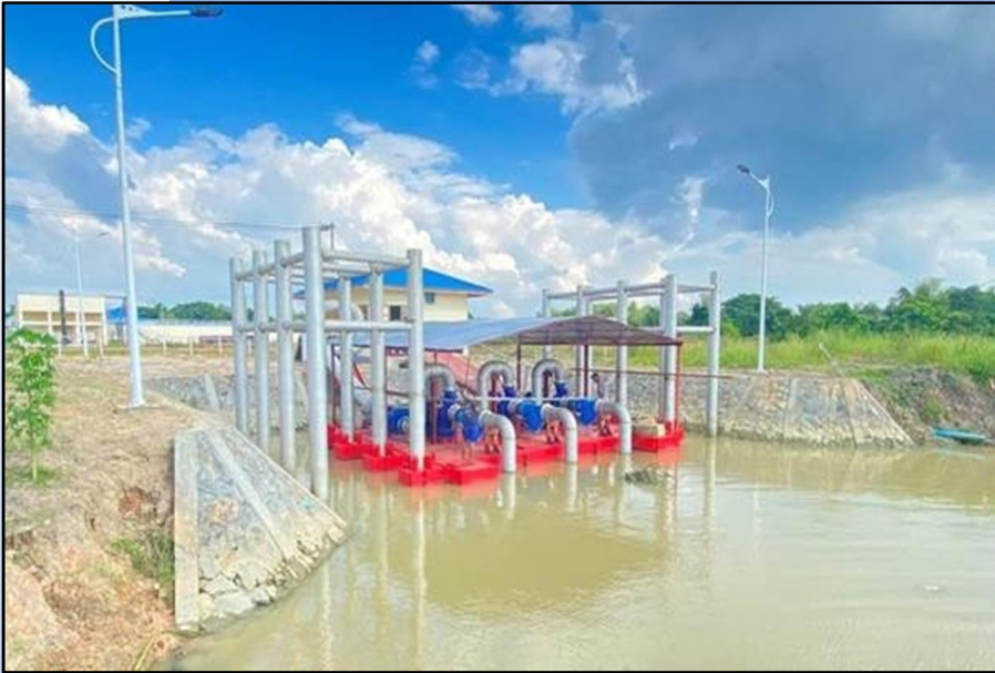
Intake structure and pontoon
