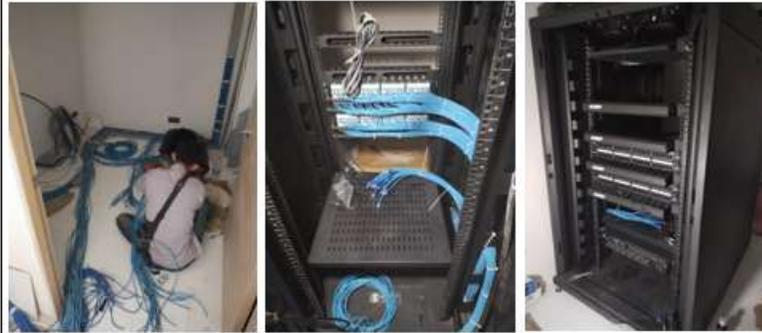
CCTV Monitor, NVR & Switch Mounting Process
