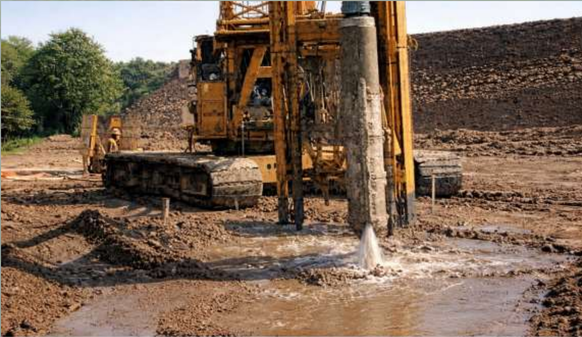
Figure 116. Vibroflotation with a water jet to assist ground penetration during construction of a vibro-replacement stone column.
