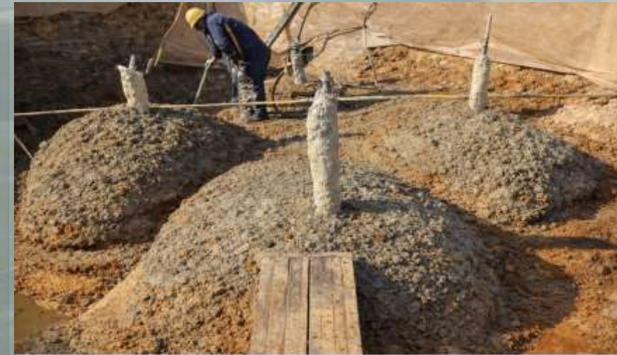
Figure 122. Soil that had been treated by permeation grouting before being exposed by excavation (Yamazaki et al. 2005).
