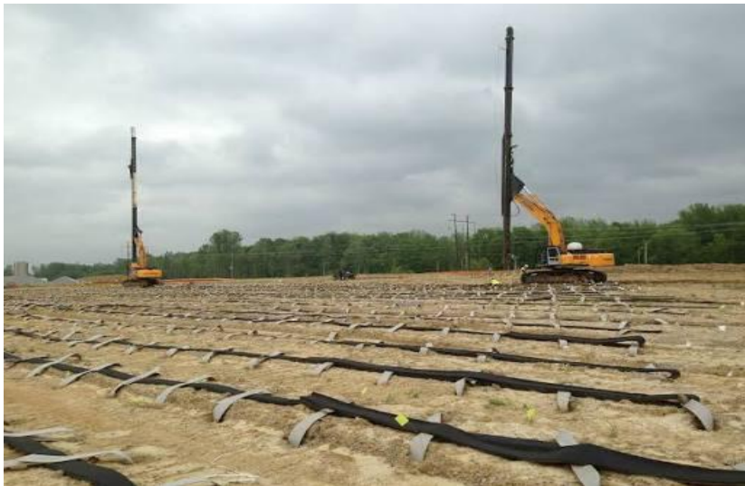
Prefabricated Vertical Drains(PVD)
