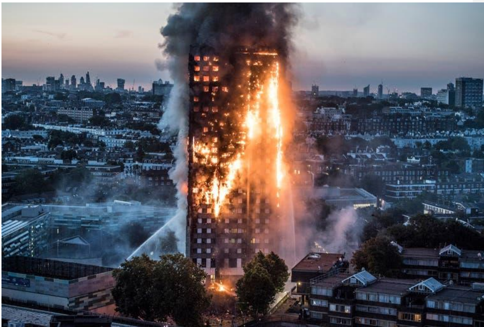
Stack Effect and Tall Building Fire Hazard
