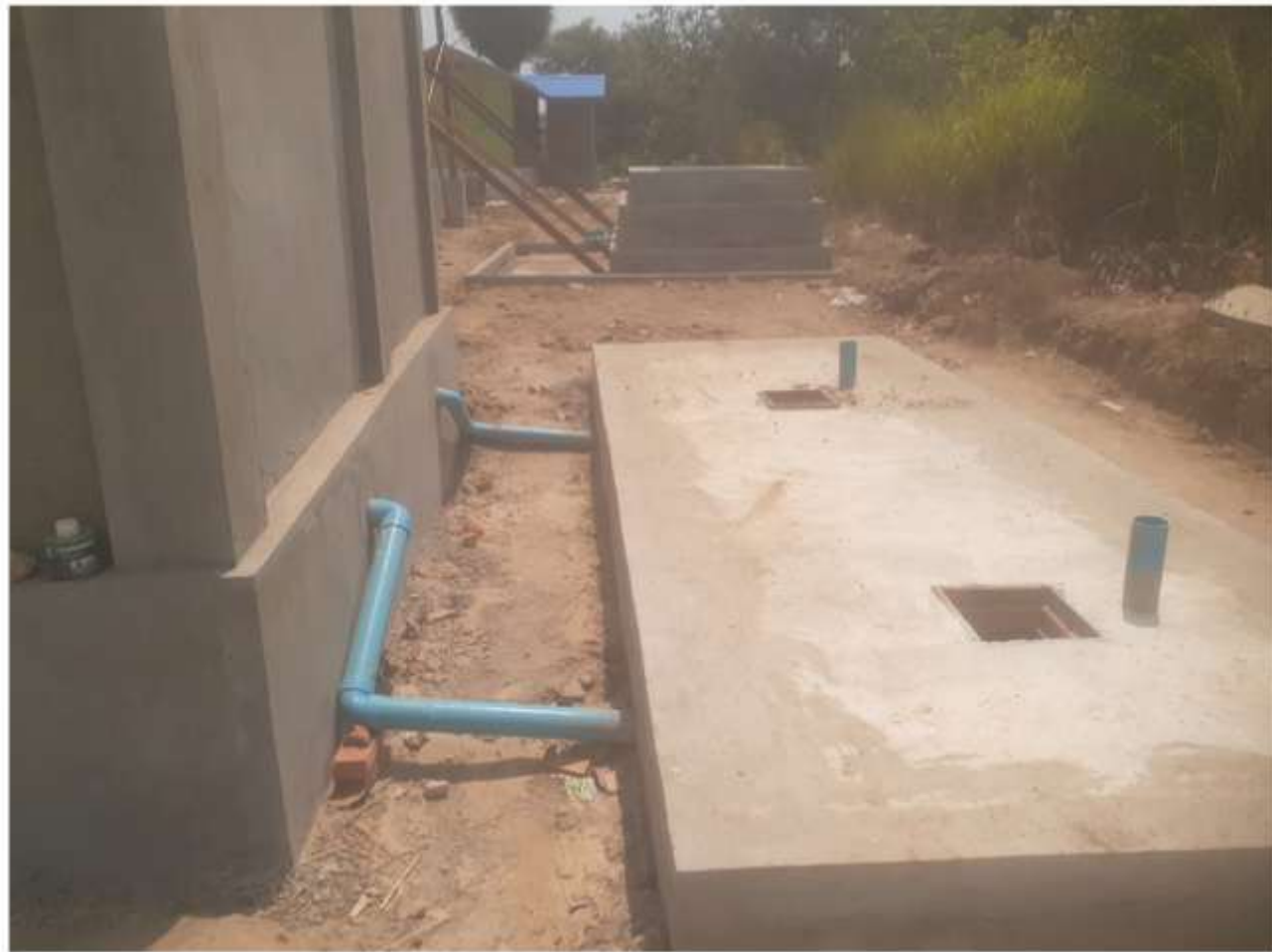
2 Units Latrine to Septic Tank Wrong Connection
