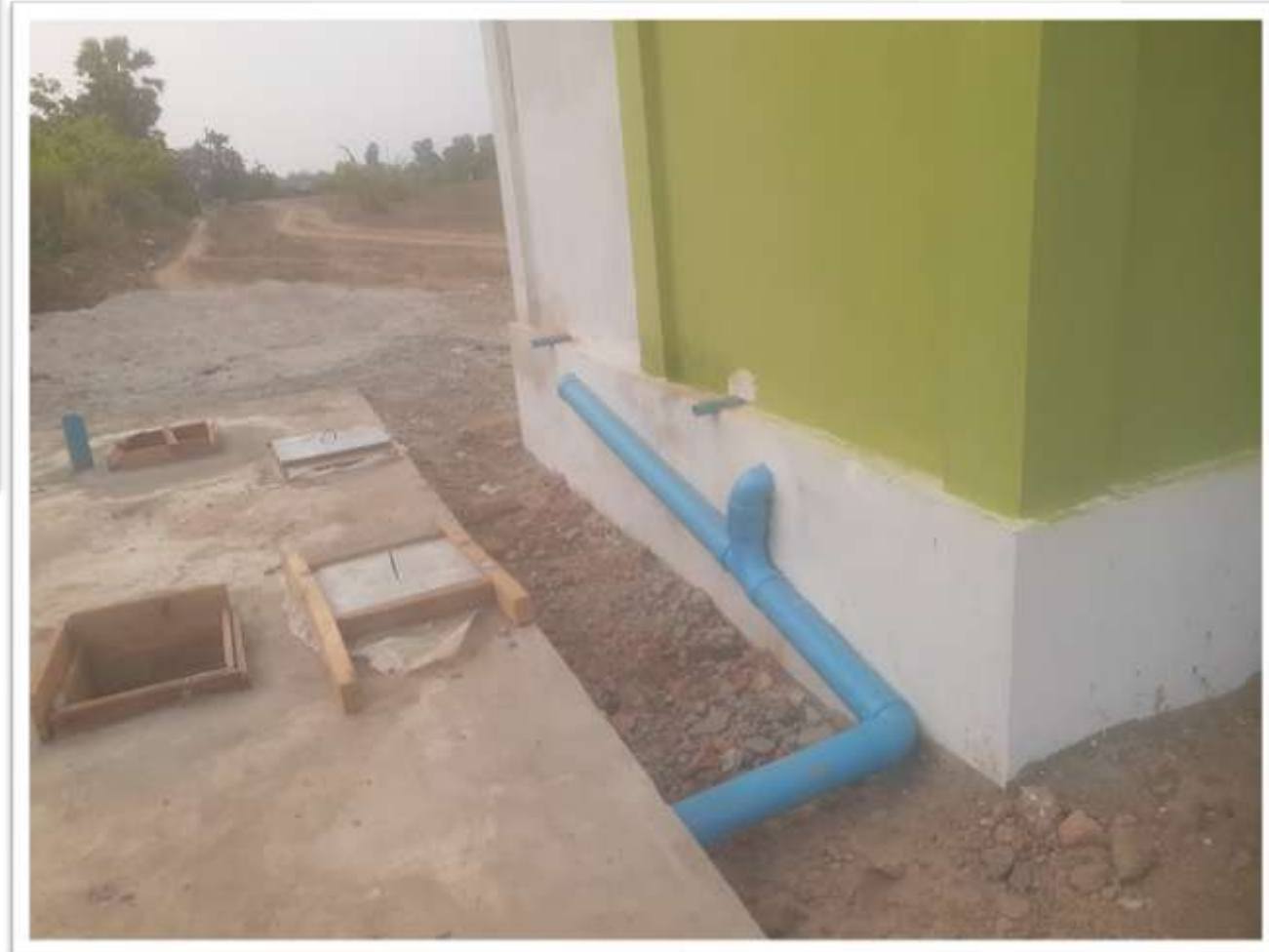
2 Units Latrine to Septic Tank Right Connection
