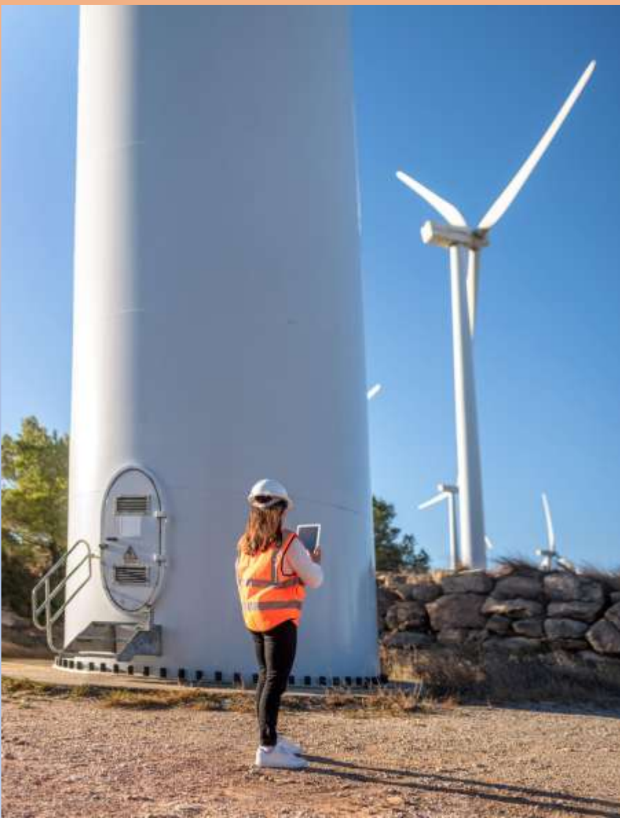
Woman Engineer. Renewable Energy Systems Engineering
