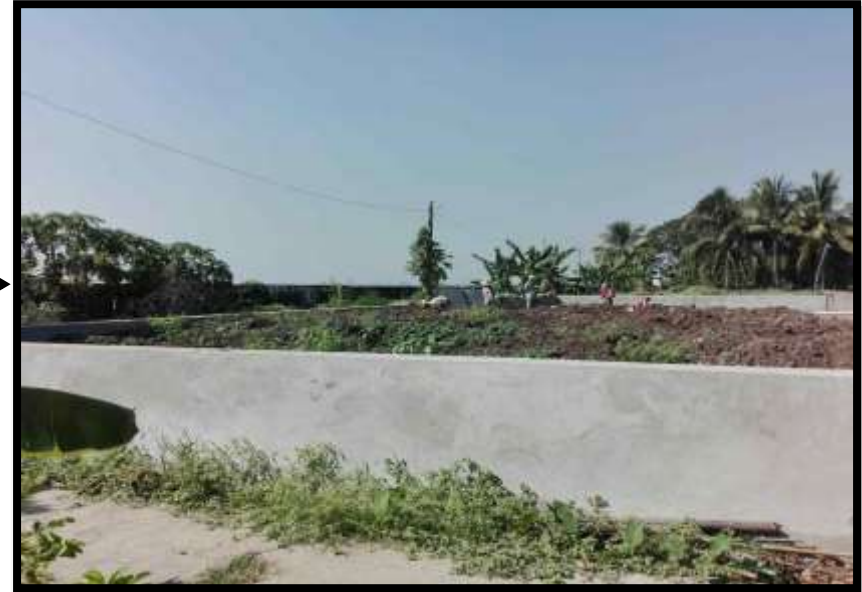
Sludge Collecting Tank
