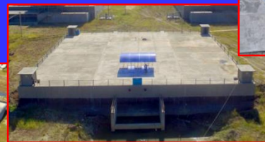
Clear Water Reservoir
