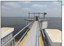
Phugyi water intake tower
