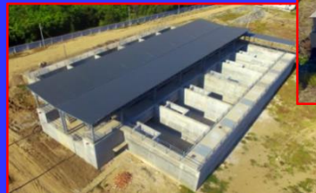
Rapid Sand Filter Basin
