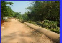
Transmission pipeline from Hlawga
