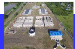
Lagunbyin WTP (on going project)
