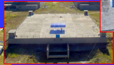
Clear Water Reservoir
