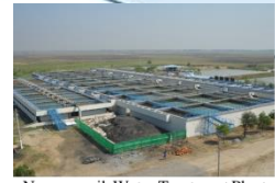
Ngamoeyik Water Treatment Plant (Nyaungnapin), 1 st phase
