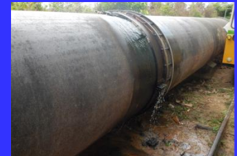
Leakages at Transmission Facilities
