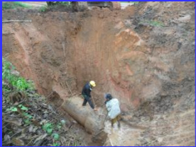
Transmission Main Breakout
