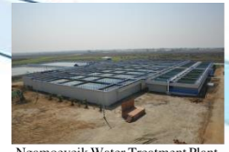
Ngamoeyik Water Treatment Plant (Nyaungnapin), 2 nd phase
