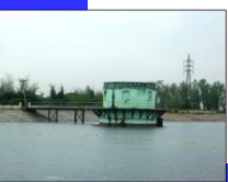
Hlawga water intake tower
