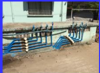
water meter installation
