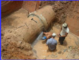
Transmission Main Breakout
