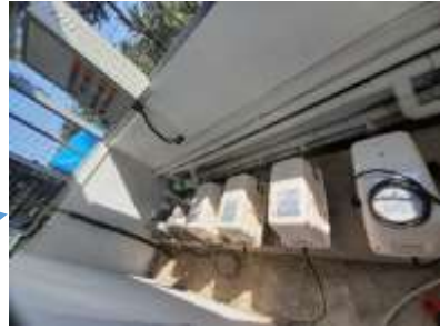
Air Blower House
