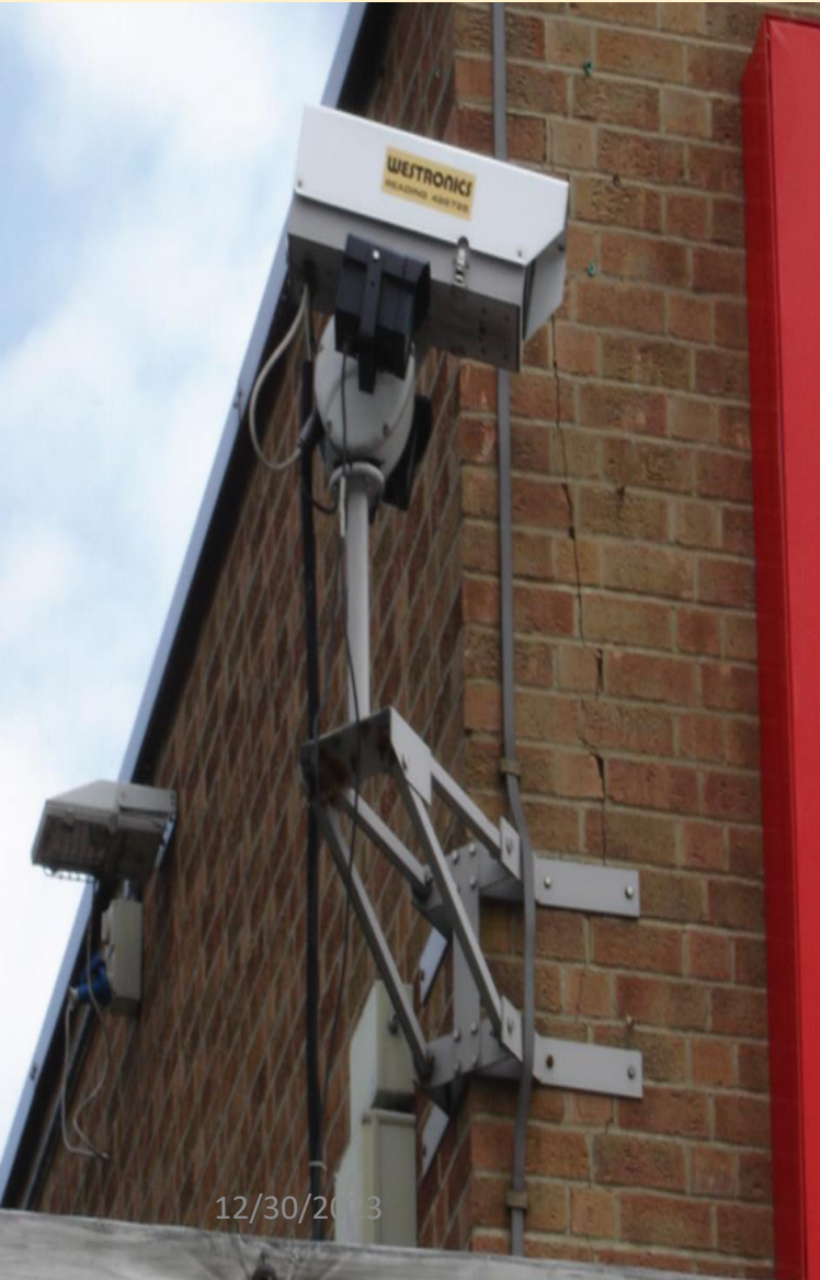
Conventional down-conductor Separation distance problem
