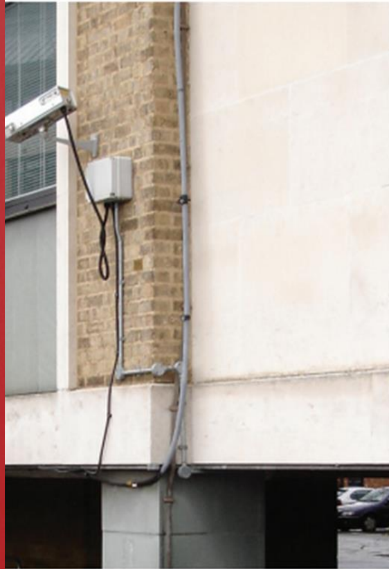
Conventional down-conductor Separation distance problem
