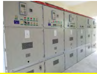
11KV 2 In 2 Out + Tie Switchgear HUYU, China
