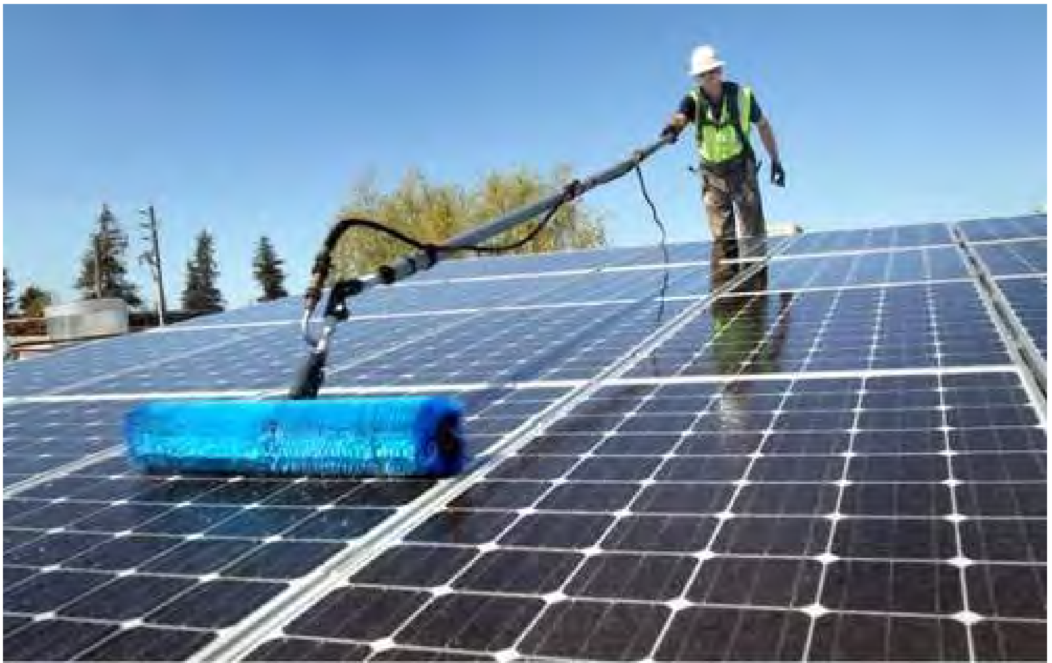
Solar panel cleaning using soft brush and deionized water
