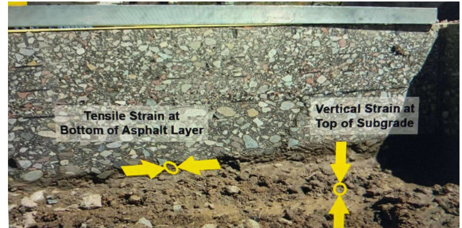
Figure 3-1. Location of Critical Strains in a Full-Depth Asphalt Pavement
