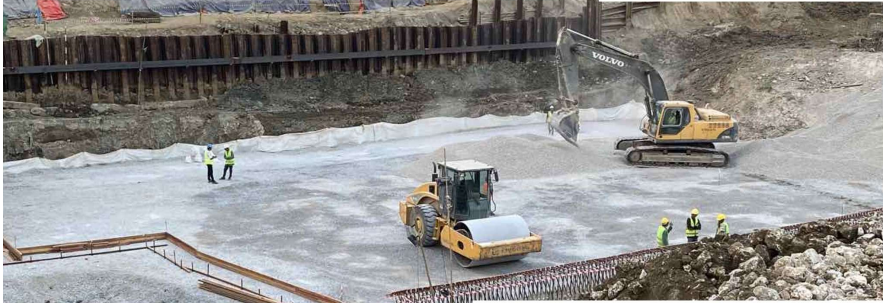
Preparation for Base Slab
