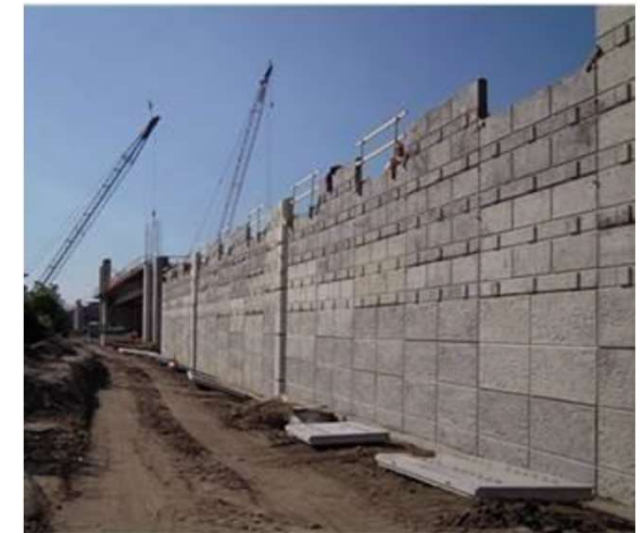
Segmental Wall at Bridge Approach road
