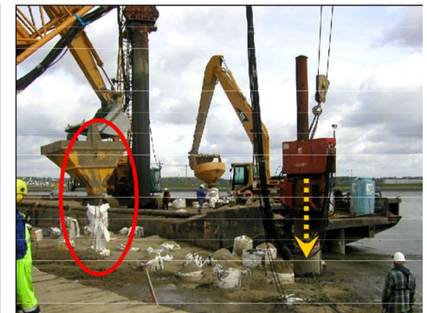
Confining capability of high strength geotextile encasement
