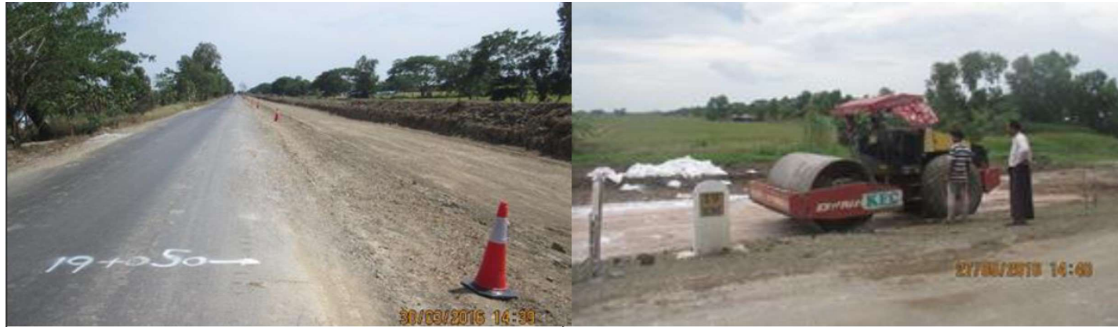
Excavation of unsuitable materials Km 19 to 22 and Lime Stabilization
