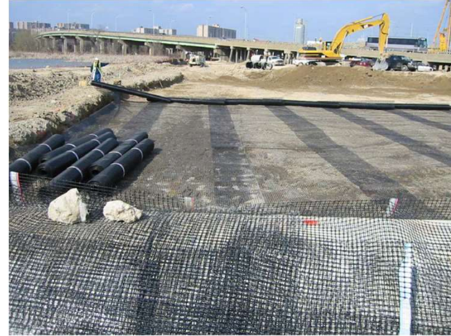
Load transfer platform reinforcement placement
