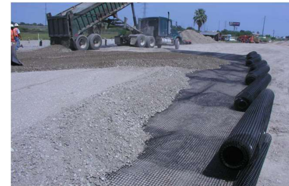
Load transfer platform select fill placement
