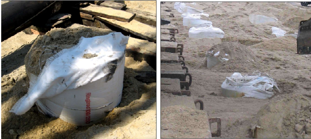
Completed Geosynthetic Encased Columns
