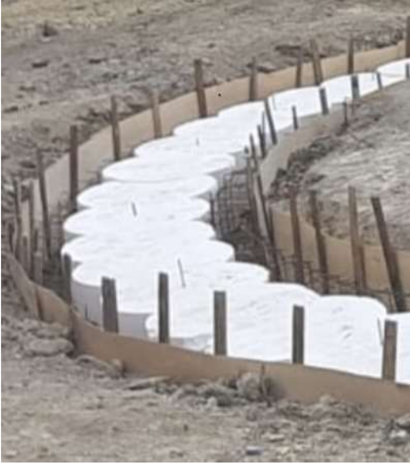
Started the Secant piling for cable tunnel shaft no-1 (3-1-2023)
