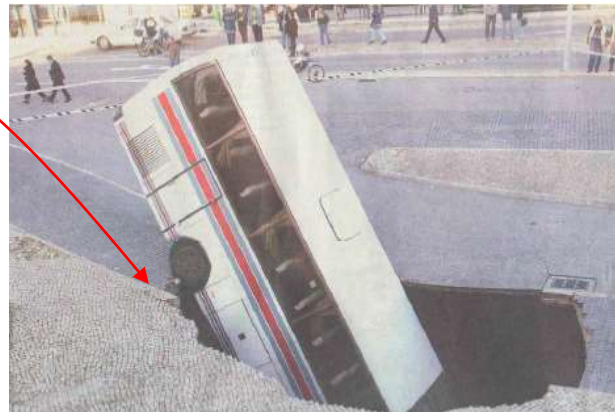
Settlement due to ground losses after tunnel construction
