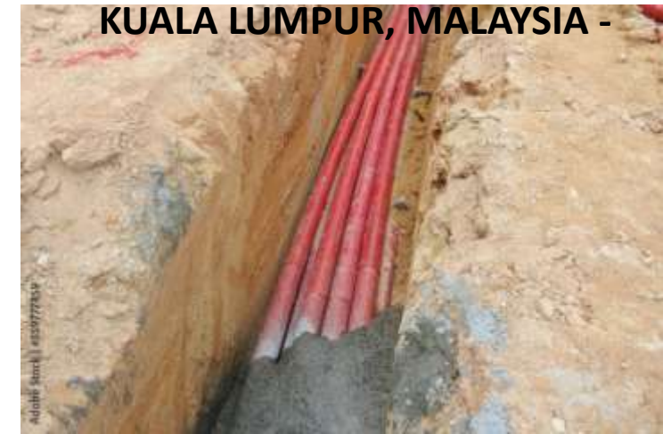
HDPE conduit pipe power conduit installed inside the ground trench
