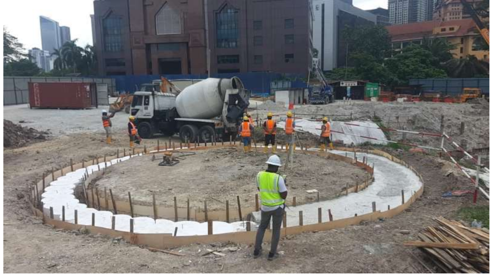
Started the Secant piling for cable tunnel shaft no-1 (3-1-2023)
