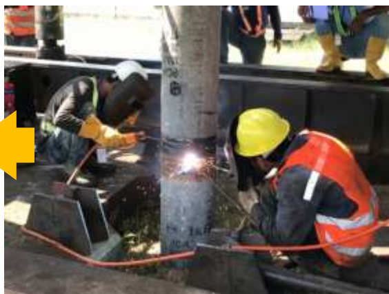
Jointing by Welding
