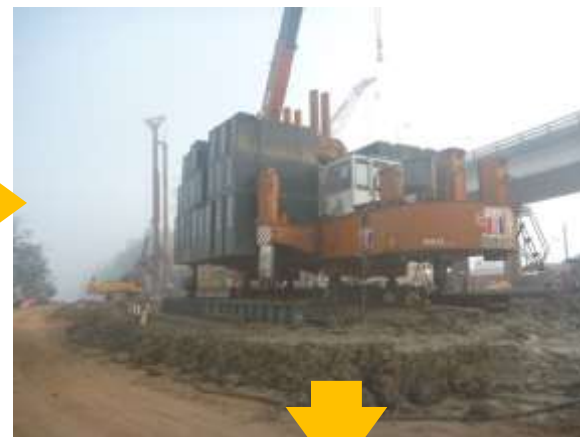
Installation of Jack-in-pile
