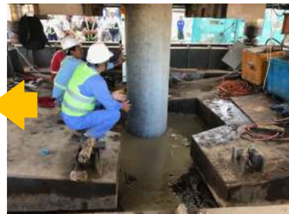
Installation of Jack-in-pile
