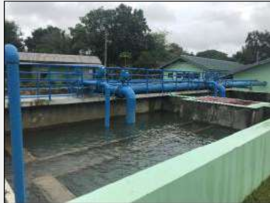
Operation of Rapid Sand Filter
