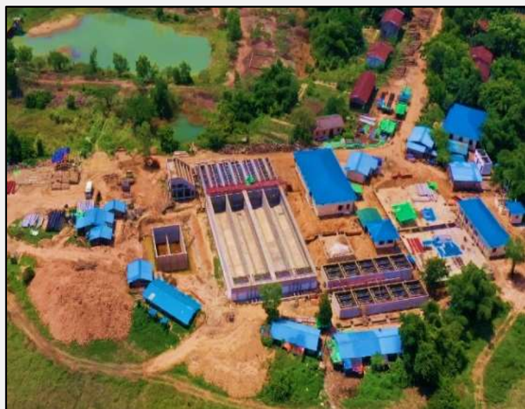
Pathein RSF Water Treatment Plant
