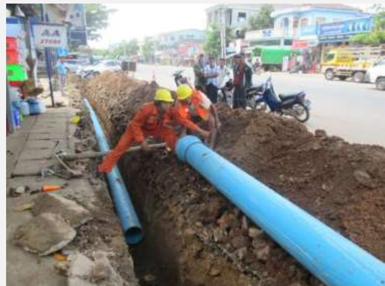
Installation of 10" PVC Transmission Pipeline
