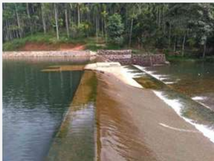
Rehabilitation intake weir
