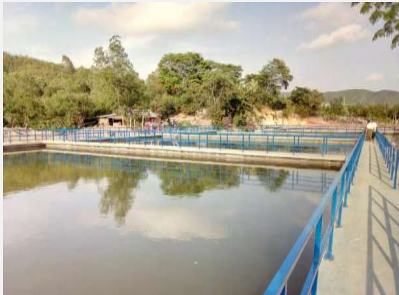
Slow Sand Filtration Facility
