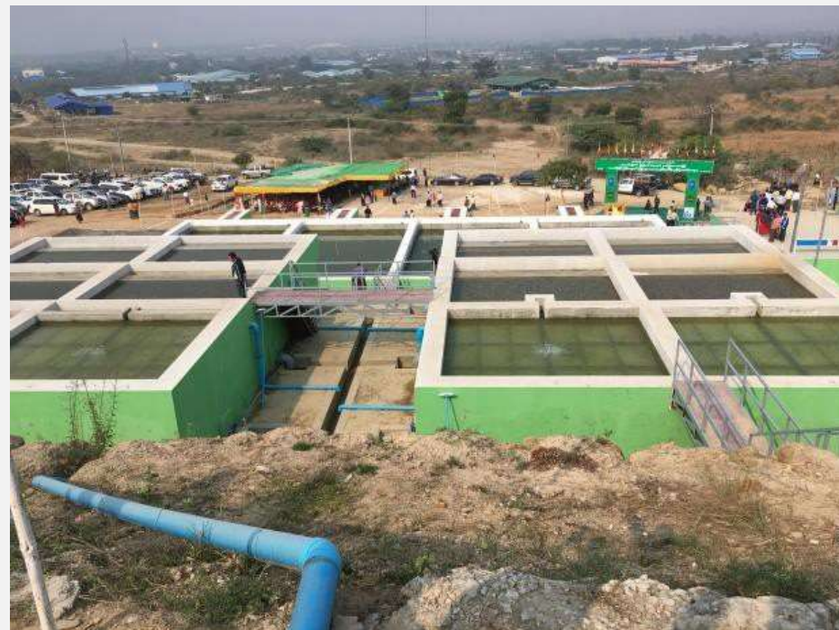
Roughing Filter and Slow Sand Filter
