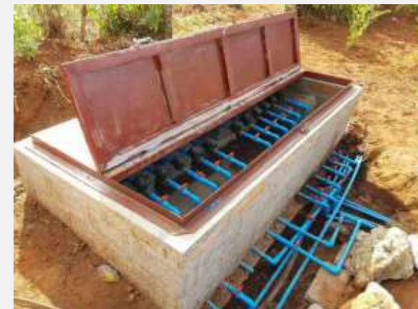
Pipe and water Installation work at net work
