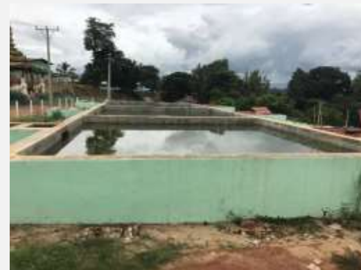
Operation of WTP
