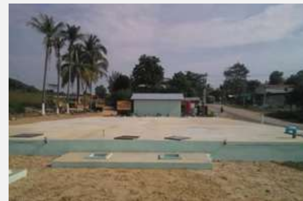
Clean Water Reservoir
