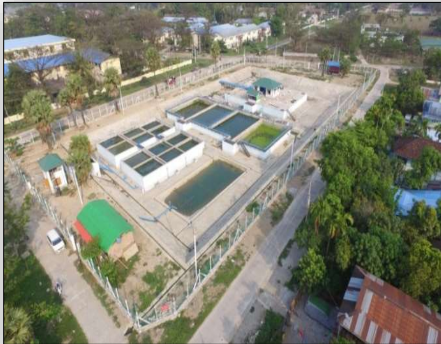
Pyapon Water Treatment Plant
