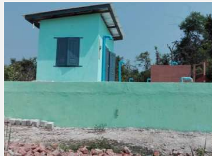
CL Dosing House and Clean Water Reservoir
