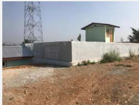
Reservoir and Chlorine Room
