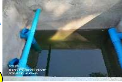
Secondary Sedimentation Tank
